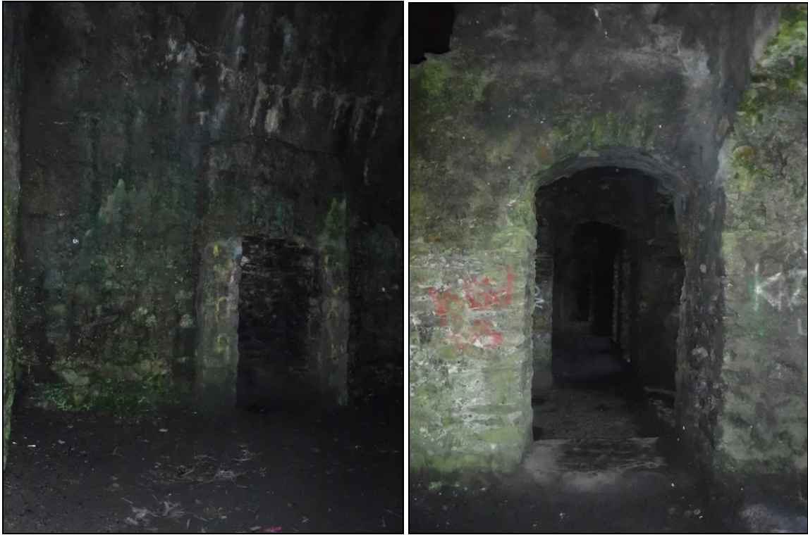
Figure 12.14 (Right) View looking west from the east room on the first floor. Note the changes in level at the door
