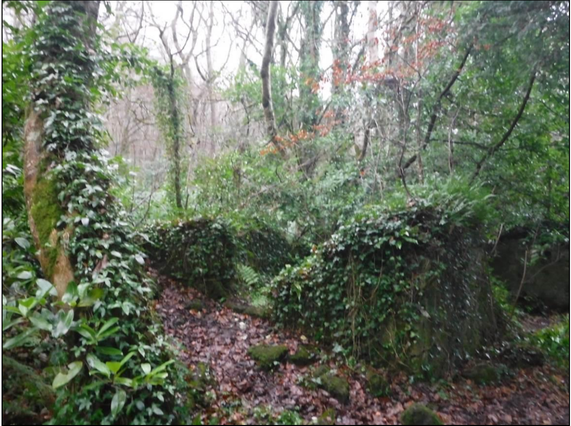
Figure 12.24 Ruined outbuilding in the Kitchen Garden
