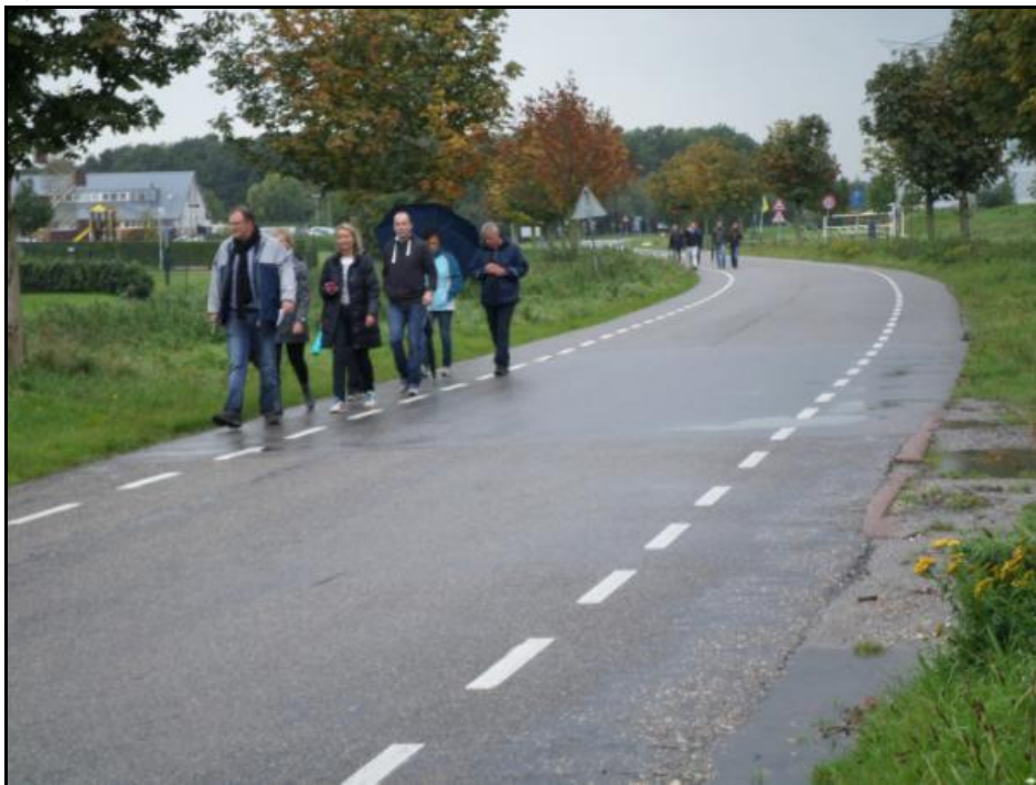
Figure 14.22 Example of a Rural Road in the Netherlands with Advisory Lanes for Pedestrians and Cyclists
