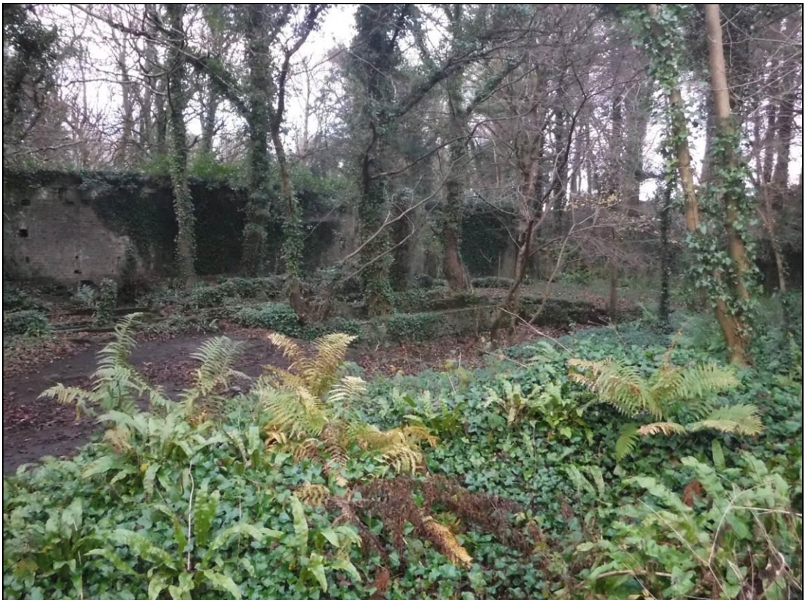
Figure 12.31 Foundations of some of the glass houses with the north and east walls of the walled garden in the background
