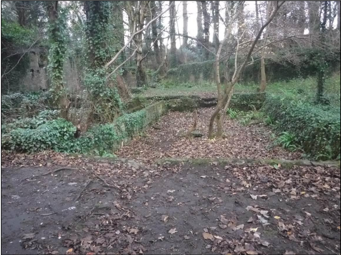
Figure 12.32 Foundations of some of the glass houses with the north and east walls of the walled garden in the background
