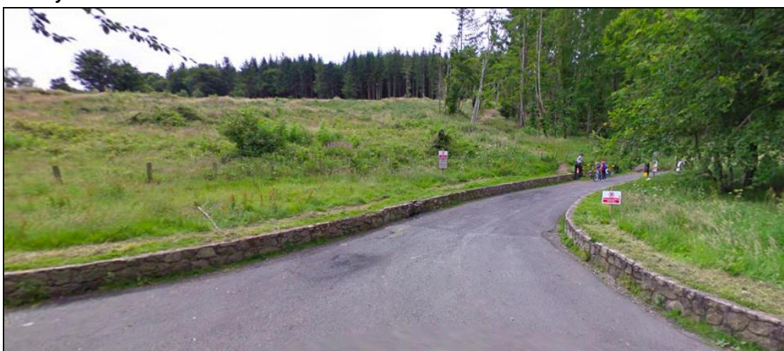
Figure 12.56 The boundary wall to the Coillte lands at Montpelier hill is by contrast a low 20 th century wall
