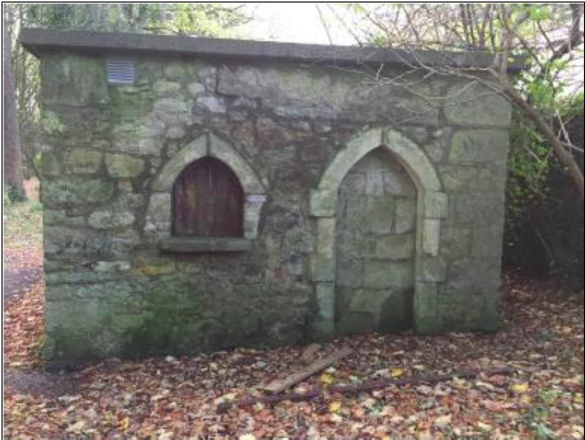
Figure 12.40 North wall of the gate lodge
