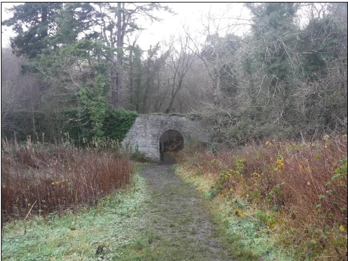
Figure 12.27 Arched entrance in the west wall of the formal garden. Note the fissure in the wall above the arch
