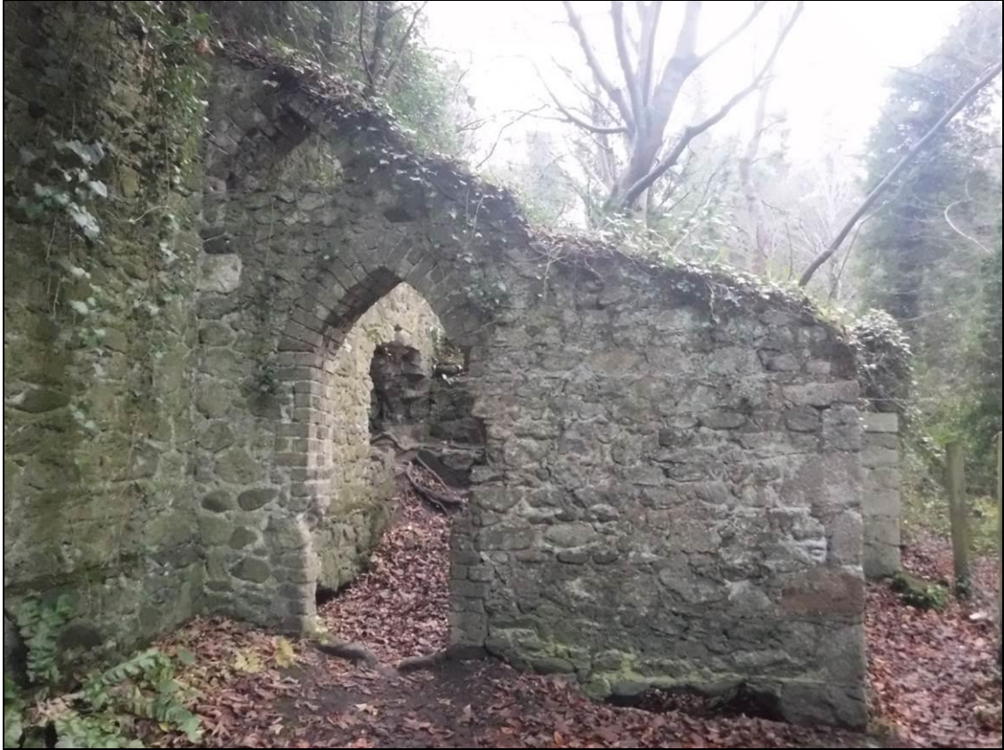
Figure 12.36 The east wall of the boiler house
