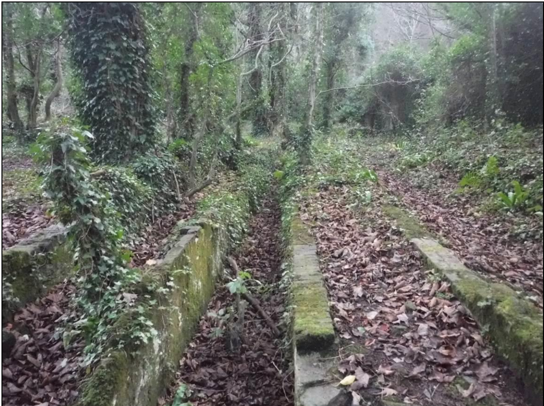
Figure 12.33 Brick foundations of some of the glass houses. Services ran in between the brick walls
