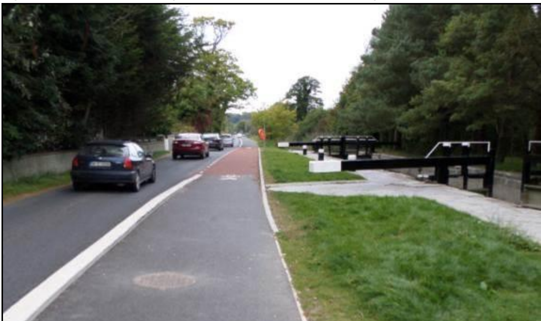
Figure 14.18 Example of Single-Track Traffic Shuttle on Oldbridge Road, Co. Meath
