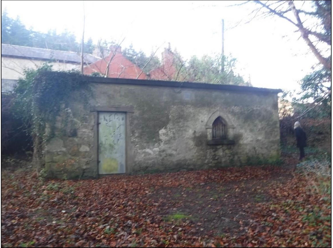
Figure 12.39 East wall of the gate lodge
