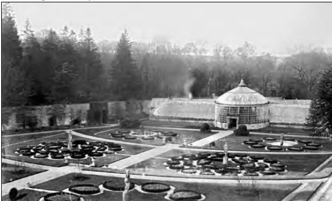
Figure 12.18 Late 19 th century photograph of the walled gardens showing the terraces and the curvilinear glass house by Turner.
