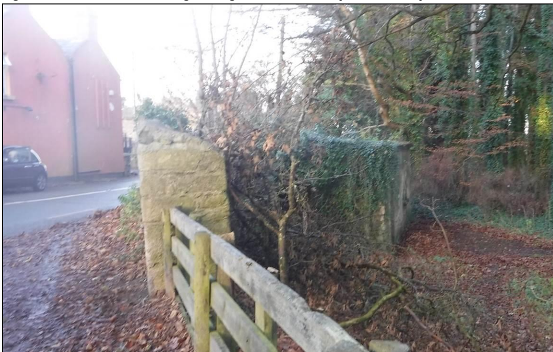
Figure 12.41 South wall of the gate lodge and the boundary wall to Massy's Wood
